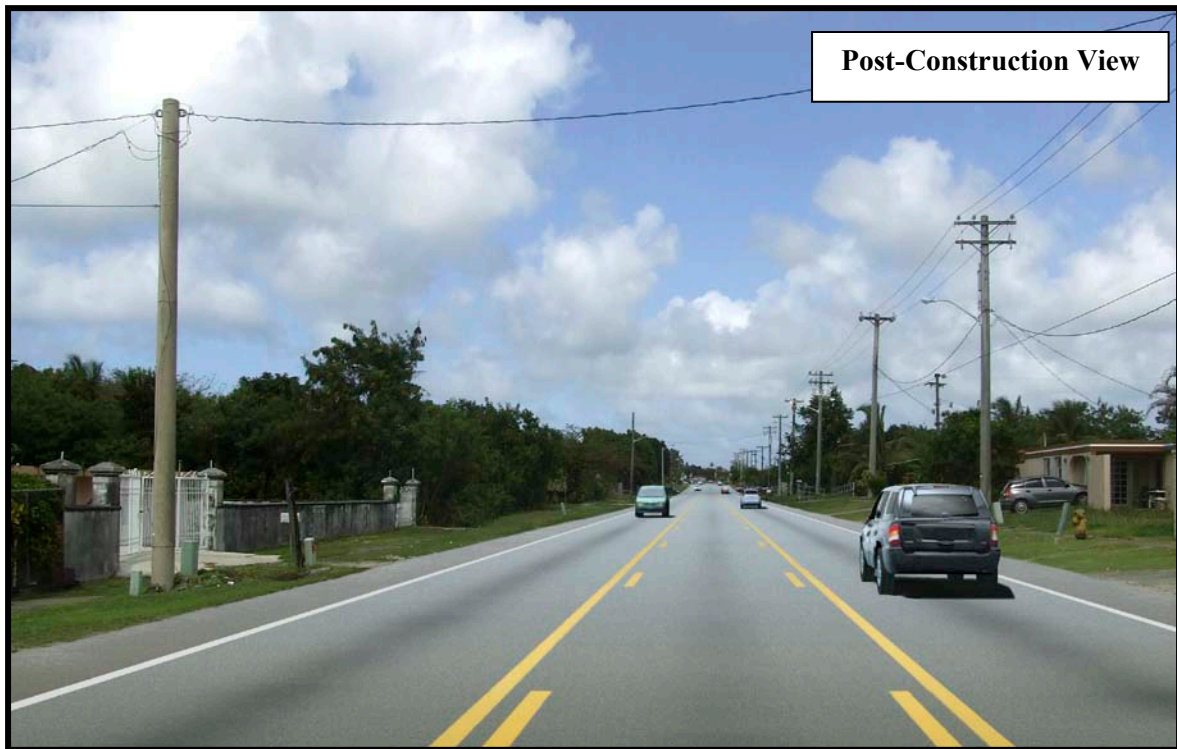
Figure 15.2-1. Key Viewpoint 1. GRN #57, Route 28 Widening
